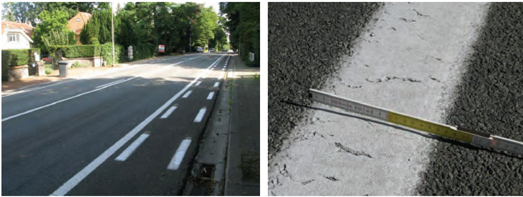
8. Measurement point MP6: N227 Mechelsesteenweg-Wezembeek-Oppem, edge line.
